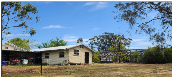
Figure 8 – Army Mess and Kitchen and Army Student Quarters.
