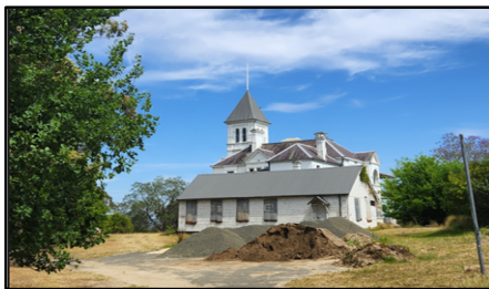
Figure 7 – Studley Park House and the Dining Hall via the southern end of the site.
