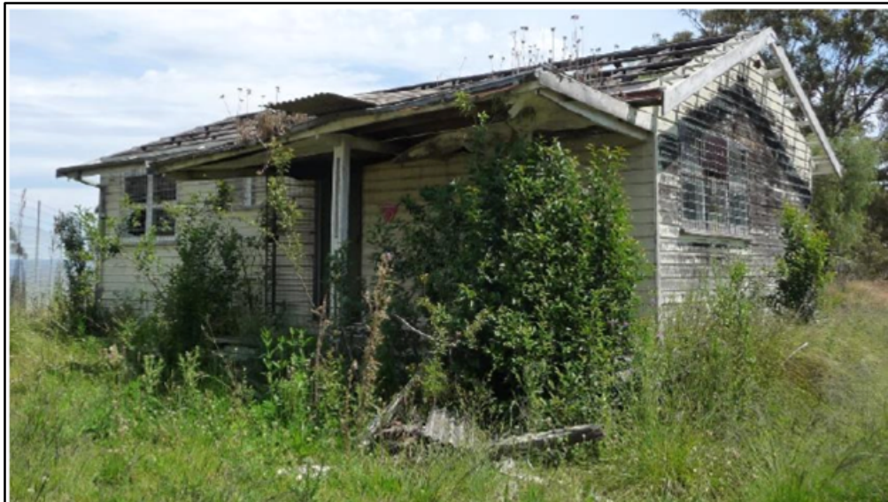
Figure 30 – Army RAP Building. Source: Figure 186 of the draft CMP.
