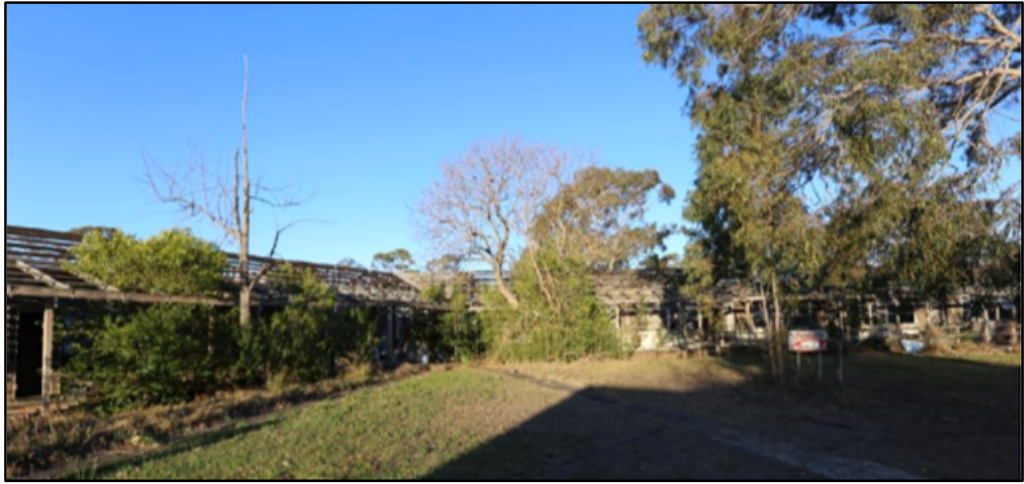
Figure 28 – Army Student Quarters. Source: Figure 174 of the draft CMP.
